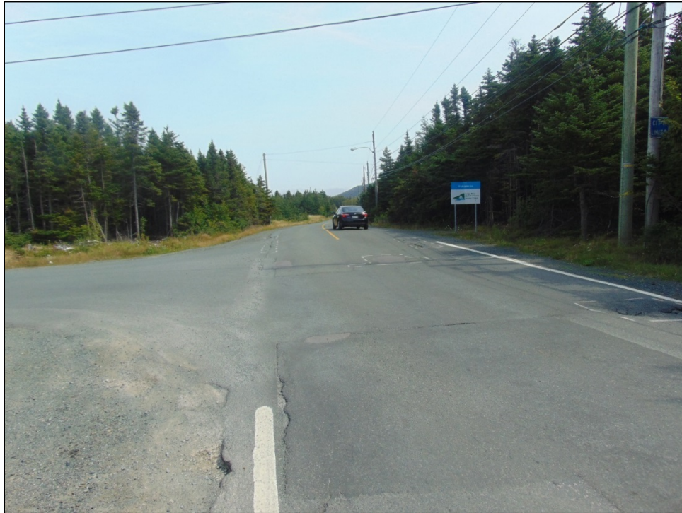
Figure 17: Pavement markings on Snow's Lane at the Town Boundary
