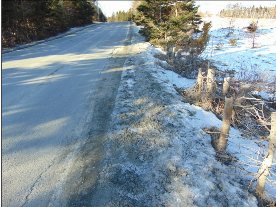
Figure 18: Varying shoulder width and condition on Snow's Lane
